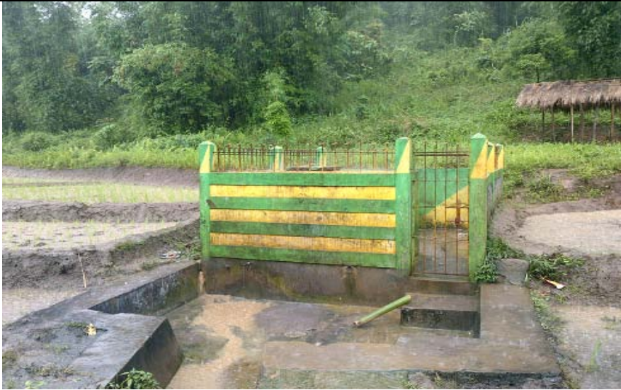
Drinking Water Tank and Footpath under RB-IWMP-IX in Ribhoi District
