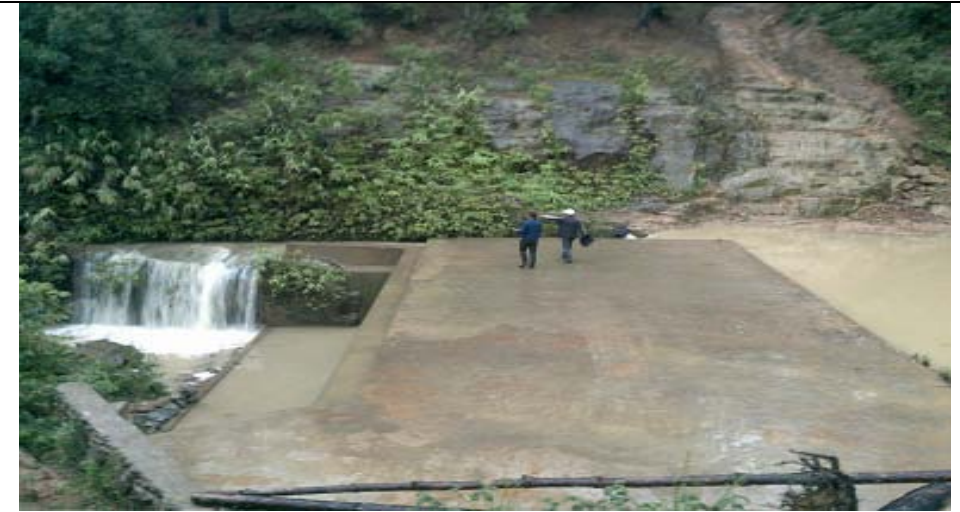
R.C..C Dam and Retaining Wall under EJH-IWMP-I in EJH District
