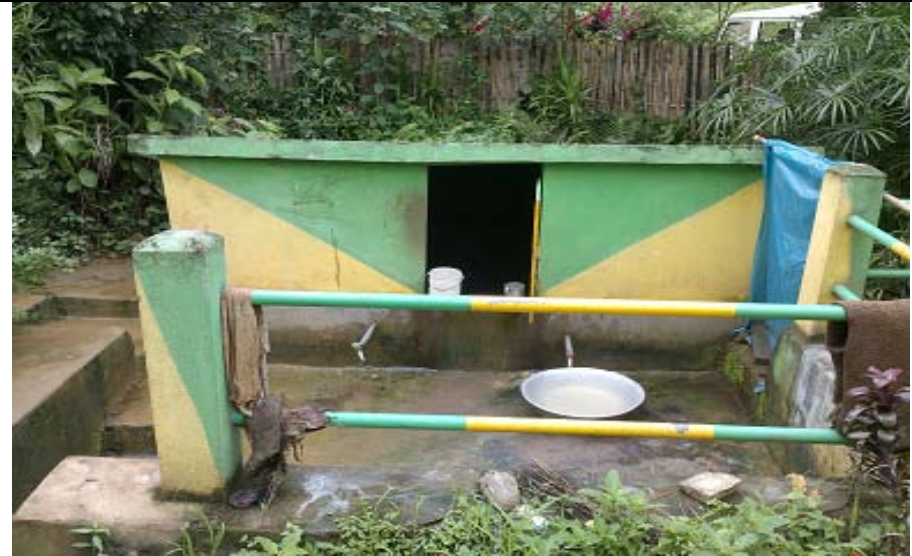
Drinking Water Tank under RB-IWMP-IX in Ribhoi District
