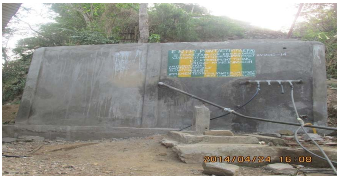
SPRING TAPPED CHAMBER WATER CUM WATER STORAGE TANK
