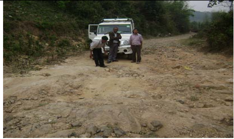
Poor Road Condition towards Project Areas under SWKH-IWMP-IV
