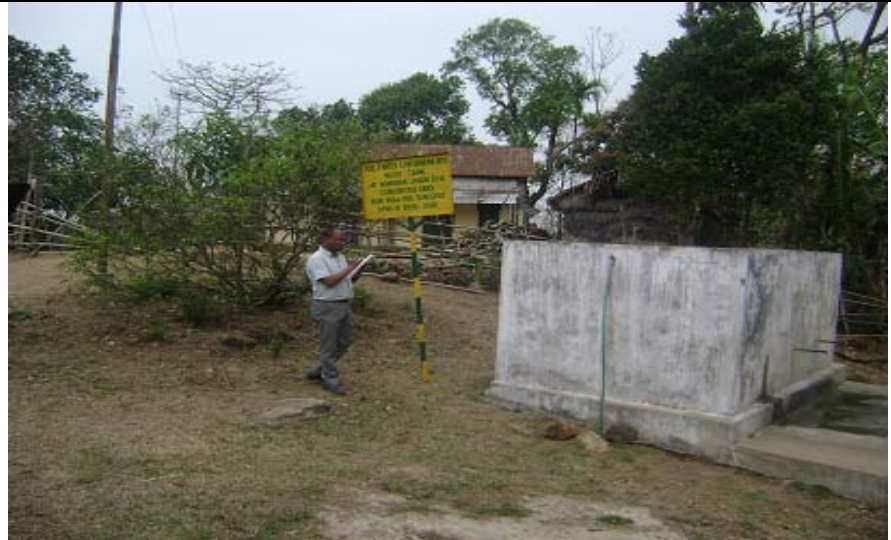
Water Tank under SWKH-IWMP-IV in S.W.K.H. District
